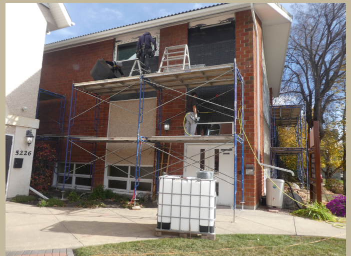
Window replacement & stucco preparation
